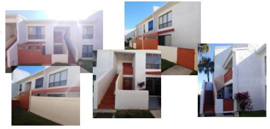
Building is approximately 85% painted. All staircases and stair rails, handrails, arbors, fencing, balcony handrails and gates, are still under construction. No abnormal, or structural concerns as of now.
